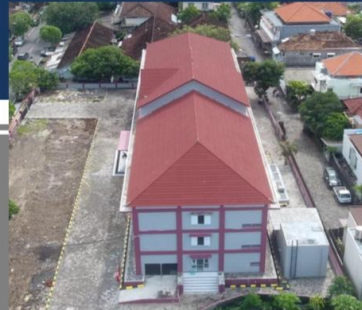
• Tampak Samping Rusun (Drone)
